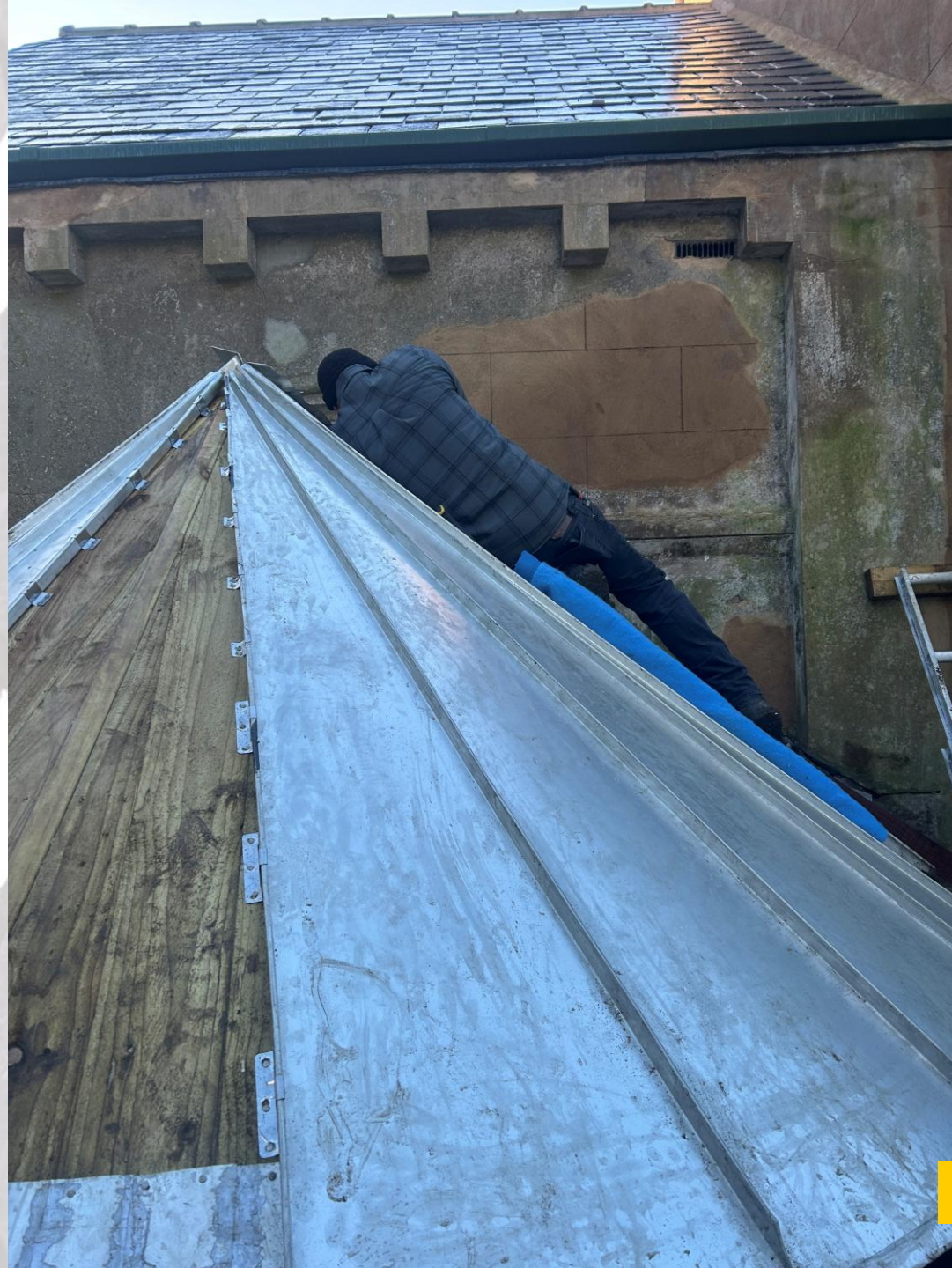
New stainless steel roof to vestry
