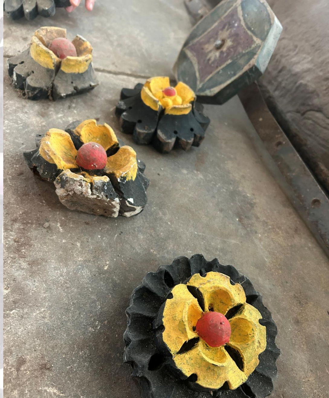
Chancel ceiling, replacing boarding where needed. Close up of bosses.
